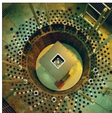
Figure 5: PROTEUS reactor core
