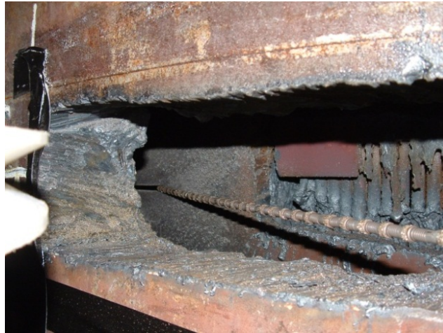
Figure 3.9: Rancho Seco steam generator cutting with a diamond wire saw
