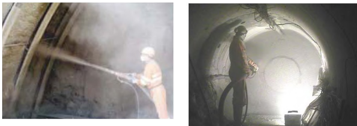
Figure 5.19: Application of low-pH cement to seal rock fractures
