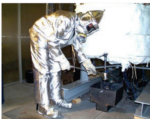
Figure 4.3. On-site melting of lead using heating blankets at the BR3 NPP
