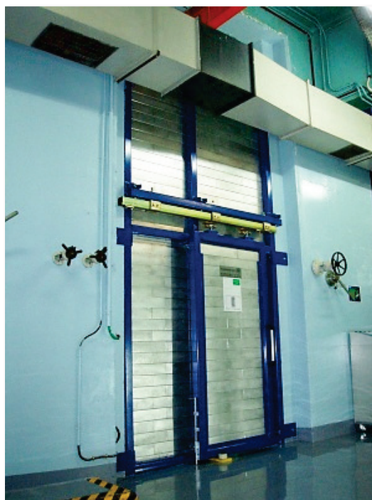
Figure 4.8. Movable shielding wall
