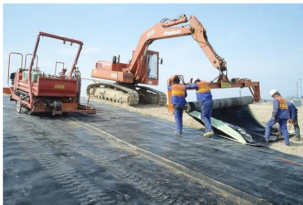
Laying a geomembrane strip. The strips are welded to each other along an axis parallel to the north-south axis.
