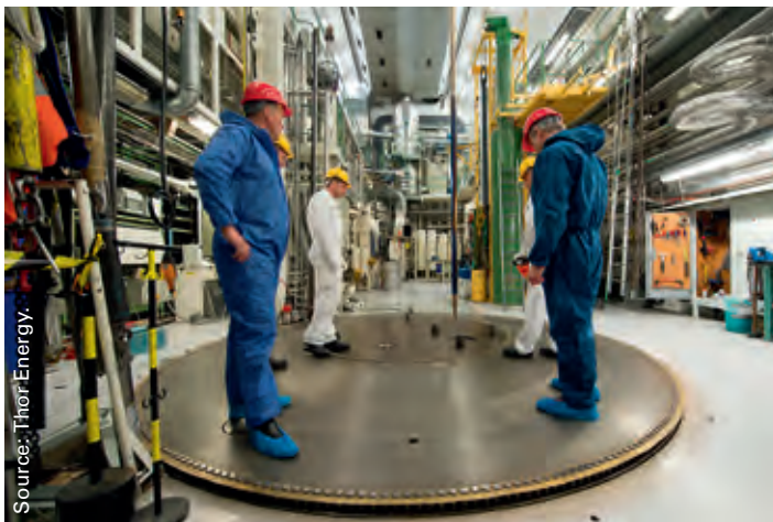
Halden reactor hall showing the rotating floor plate above the cavity containing the reactor vessel, Norway.
