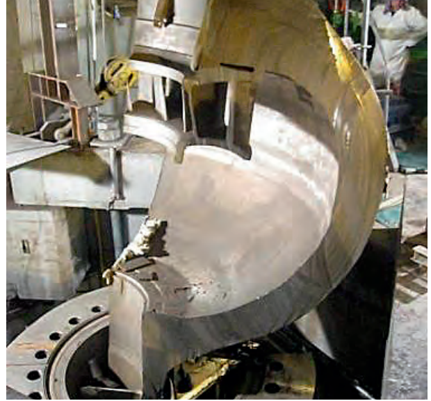
Dismantling of elements from the primary pump, José Cabrera nuclear power plant, Spain.
