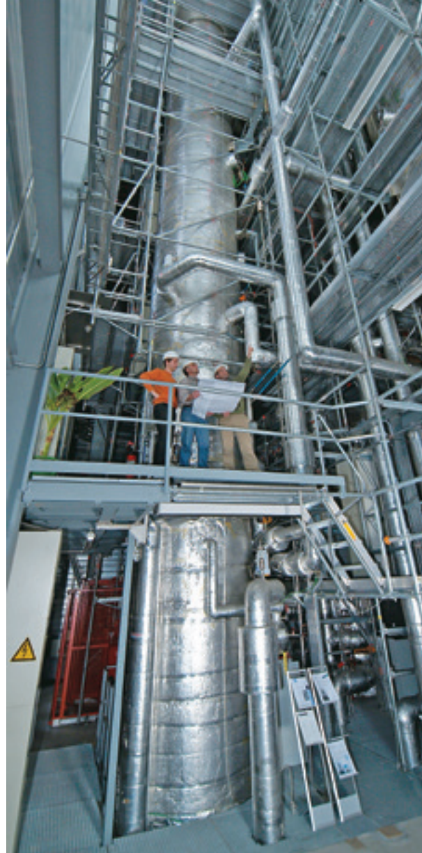
PANDA, a large-scale thermal-hydraulics test facility. Paul Scherrer Institute, Switzerland
