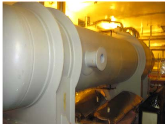
P8: RHRS - Heat exchanger
