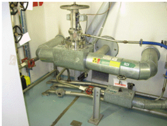
P3: CVCS - Non regenerative heat exchanger
