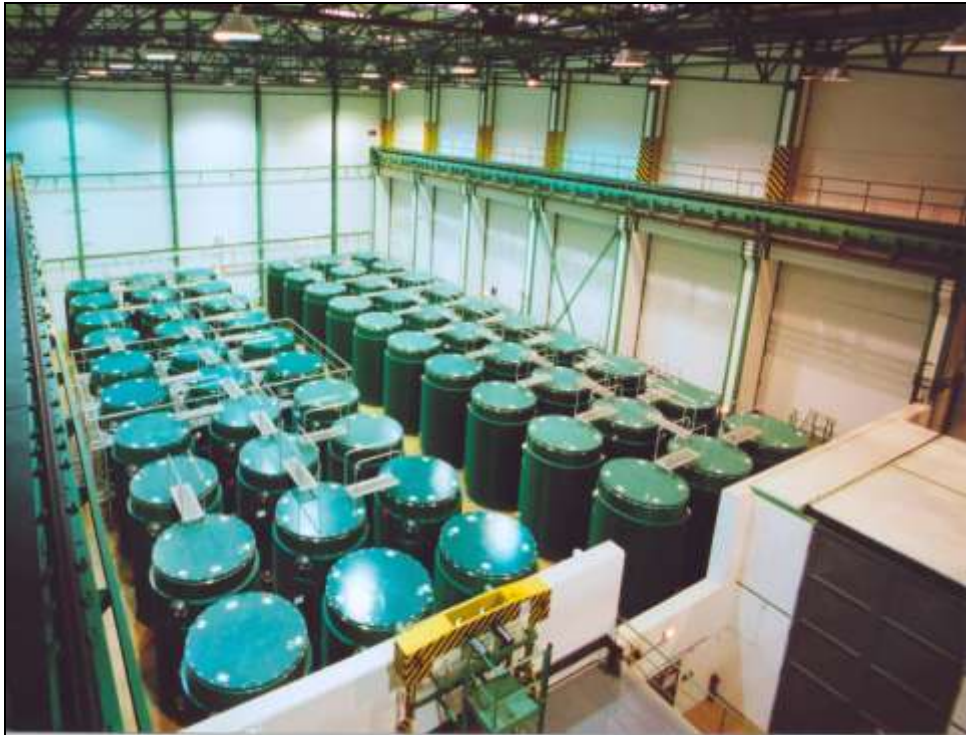
Fig. 4.2 Storage hall of ISFSF Dukovany
