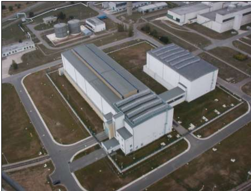
Fig. 7.1 View of SFSF Dukovany (left) and ISFSF Dukovany (right)
