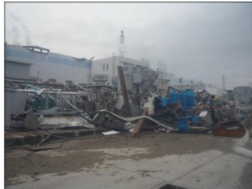
Unit 3 Sea Pump Area
