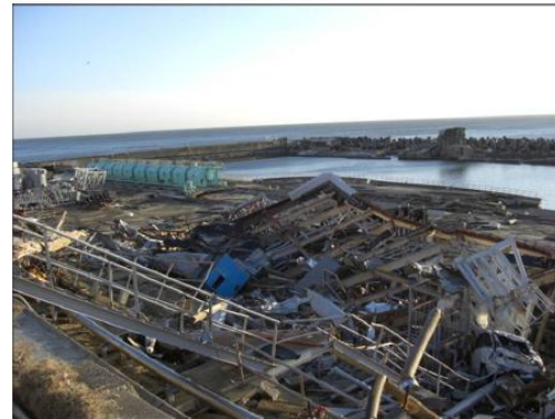
Unit 5,6 Intake Screen Area
