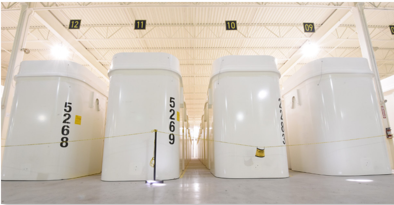
Figure 3.6. Spent fuel dry storage containers in Canada
