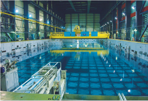
Figure 3.1. Spent fuel wet storage in France and Sweden
