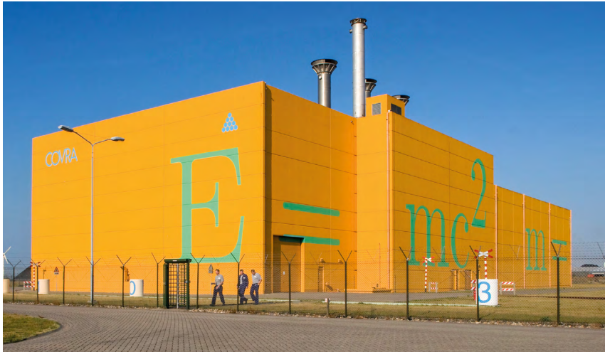
High Level Radioactive Storage and Treatment Building.
