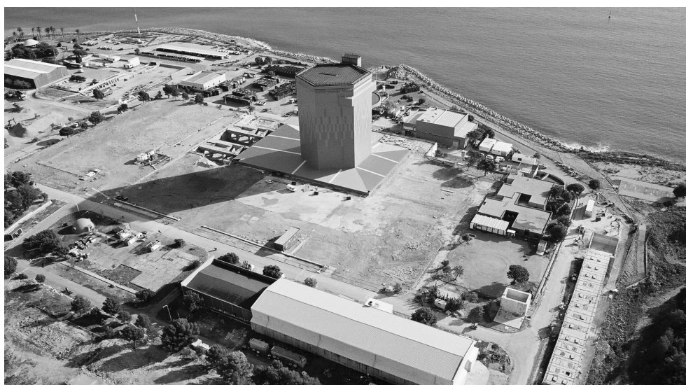
Figure 2. Vandellós-I, safe enclosure, at the end of the level 2 decommissioning works, May 2003
