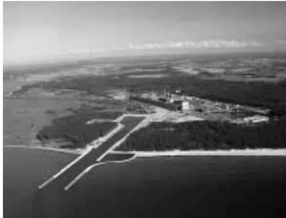
Figure 33: Greifswald Nuclear Power Plant
