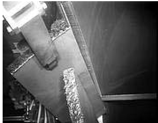
Figure 44: Removing a cut segment
