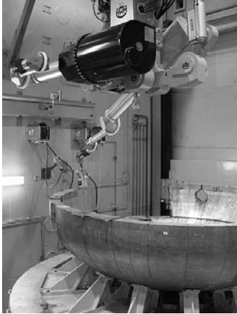
Figure 37: Dismantling of activated components – control station
