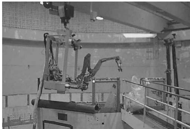
Figure 9: suspended carrier. Dual Arm Work Platform at CP-5
