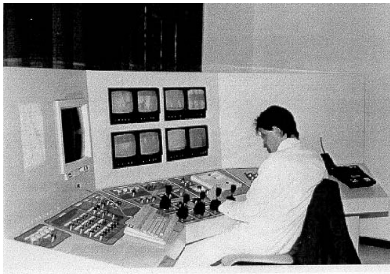
Figure51: ATENA machine control room
