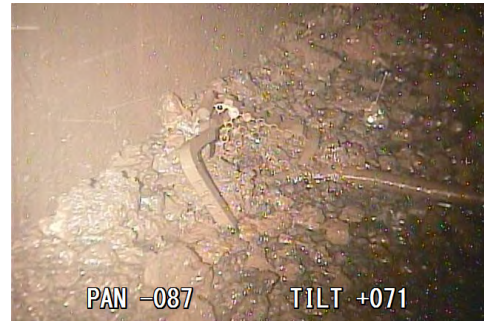
Fuel debris inside the primary containment vessel in the Unit 2 reactor building at the Fukushima Daiichi Nuclear Power Plant (fuel debris is a substance that has cooled and re-solidified while being mixed with various materials after the fuel in the reactor melted as a result of the accident). The image was captured by a remote-controlled camera attached to the tip of a survey device. Source: TEPCO Holdings
