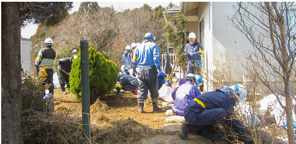
Workers decontaminating a residential garden in Okuma Town (photo taken in March 2016). Source: Decontamination archive site, http://josen.env.go.jp/archive/detail/?OK-01-P0022
