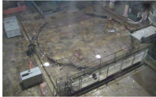
The refuelling floor on the upper part of the Unit 2 reactor building at the Fukushima Daiichi Nuclear Power Plant. Due to contamination by radioactive substances, the situation is being stabilised using remote-controlled heavy machinery and robots. Source: TEPCO Holdings
