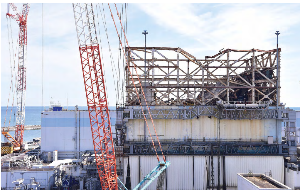
State of the Unit 1 reactor building at the Fukushima Daiichi Nuclear Power Plant (photo taken in March 2021). After a large cover is installed over the top of the building and rubble is removed, it is planned to start fuel removal in the spent fuel pool in the fiscal years 2027 to 2028. Source: TEPCO Holdings
