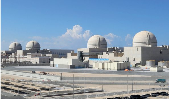
Barakah Nuclear Power Plant, United Arab Emirates.
