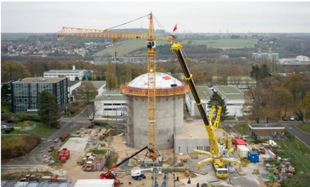
Figure 1. Picture of the VeRCoRs mock-up – External dome positioning, 11 December 2015
