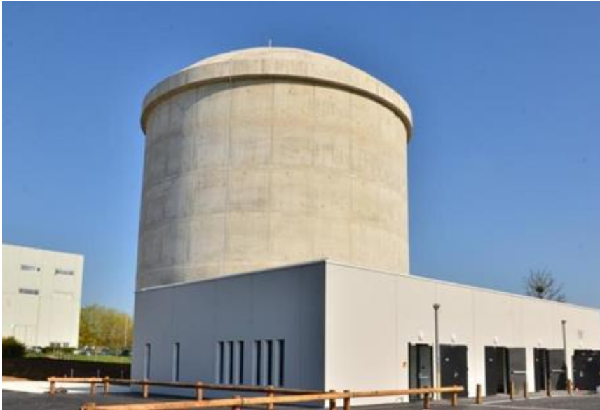
Figure 2. Picture of the completed VeRCoRs mock-up, 4 August 2016
