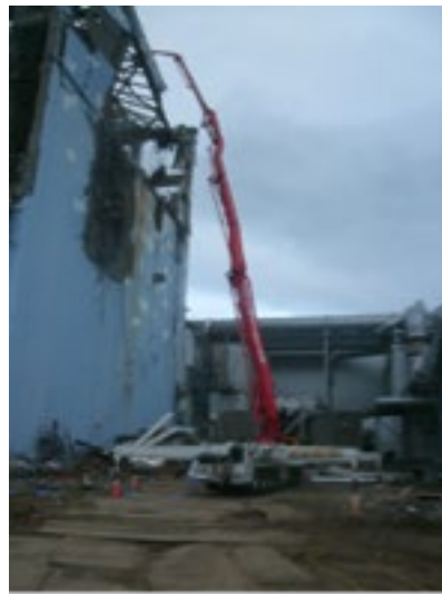
Figure E.1.11. Remote water injection by concrete pump truck
