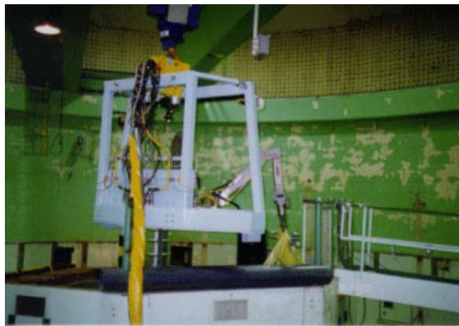
Figure B.14. DAWP Used for material handling in a high radiation area
